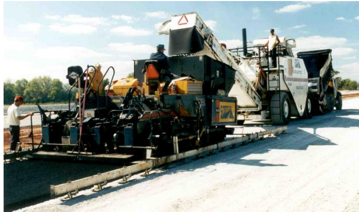
Figure 2-11. Example of Material Transfer Device.
