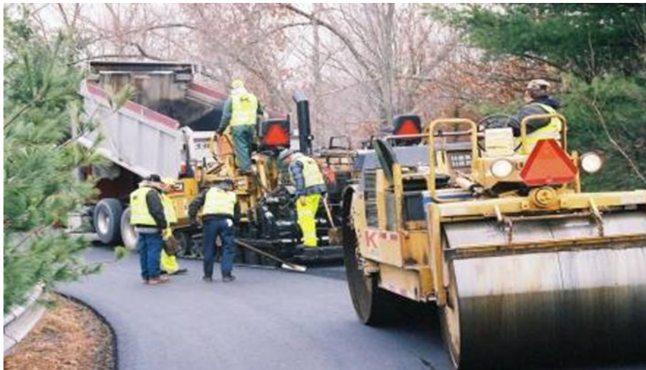
Figure 2-10. End Dump Truck Discharging Mix into Paver.
