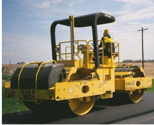
Figure 2-13. Vibratory Asphalt Compactor.
