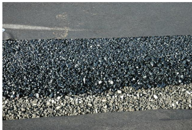
Figure 7-1. Typical Porous Pavement Design.
