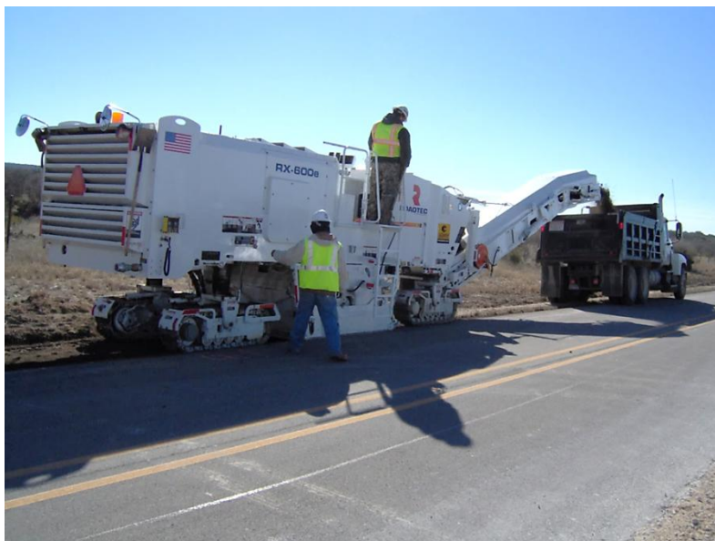
Figure 9-3. Cold Milling.
