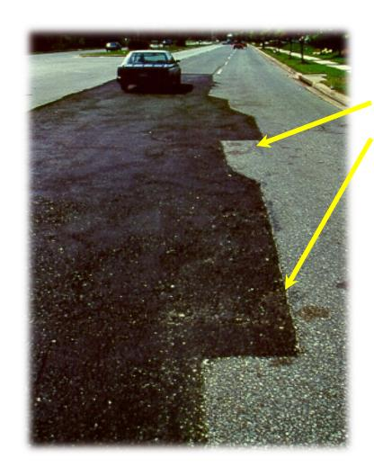
Irregular patch - getting proper compaction is going to be difficult on this one.
