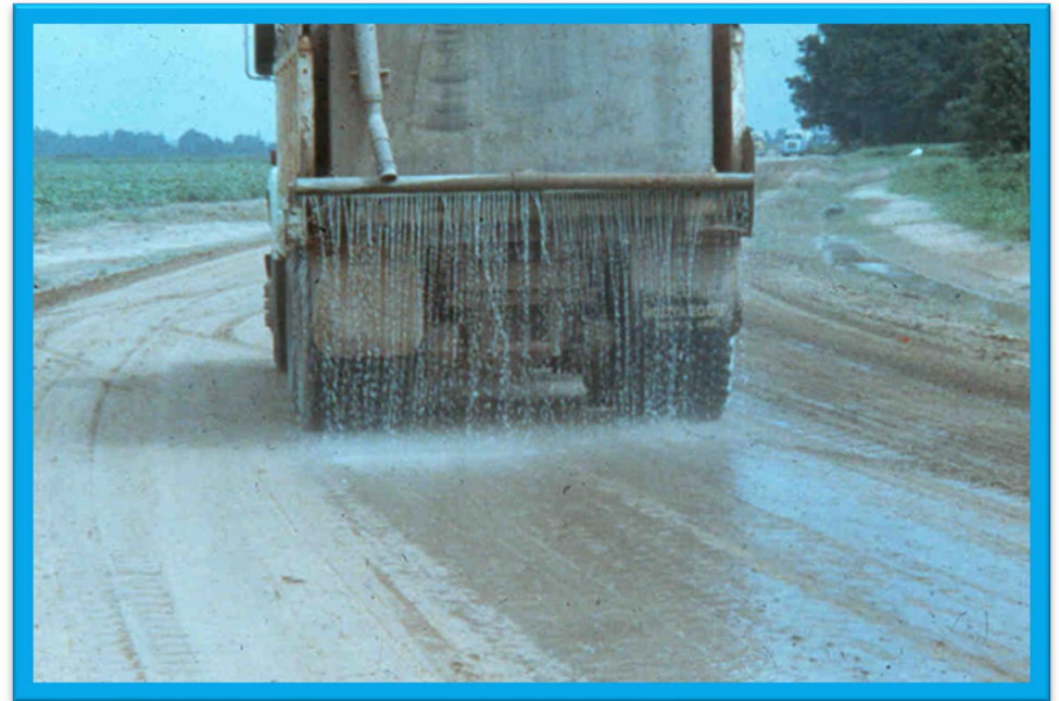
Moisture Cured Subgrade
