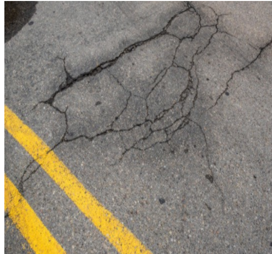
Cracking
