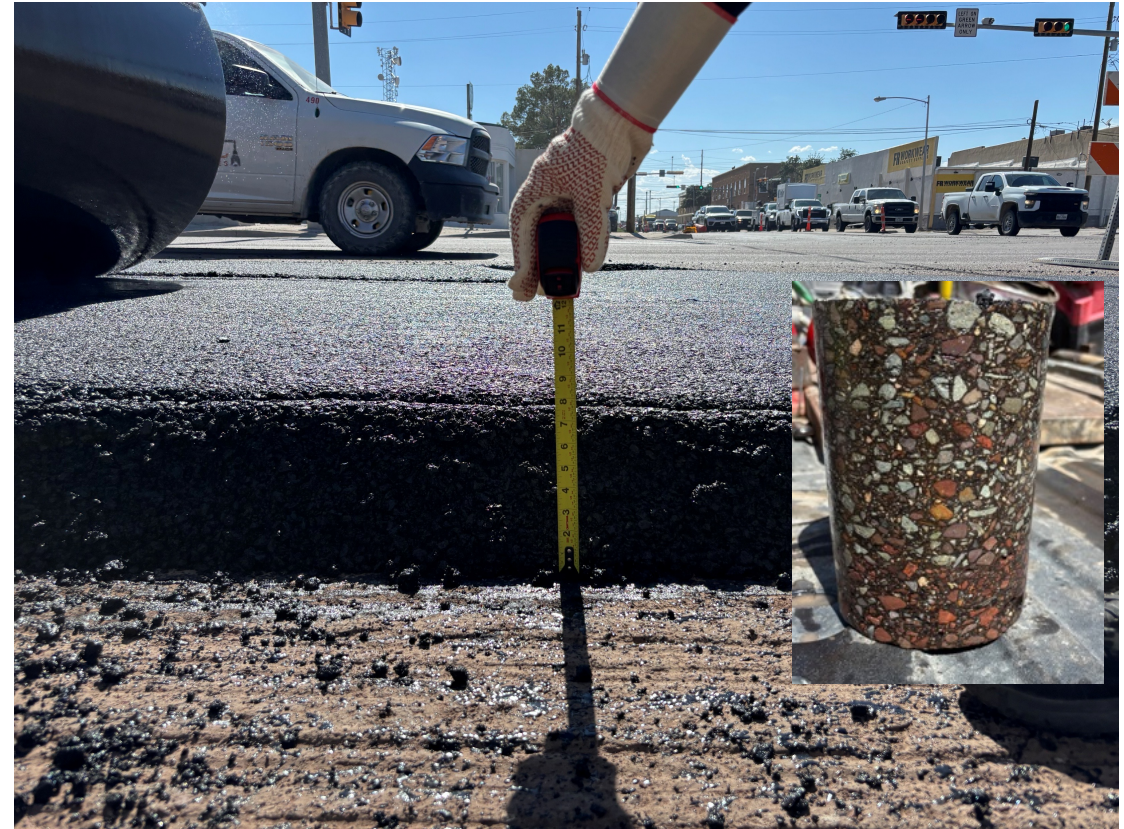
6 inch thick lift paving
